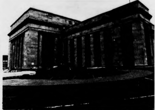
Amtrak's 30th St. Station
